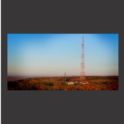
Self Supported Communication Towers
